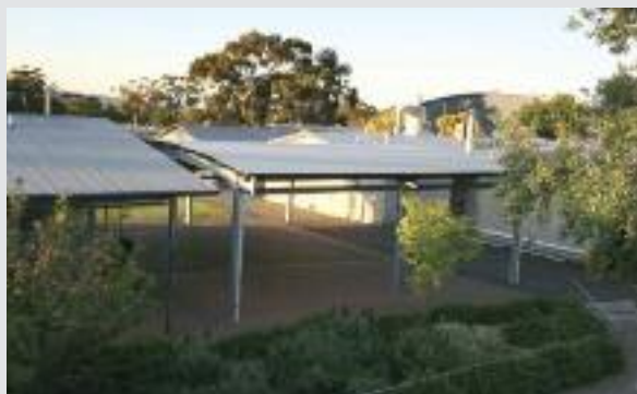
Curved roof over courtyard
