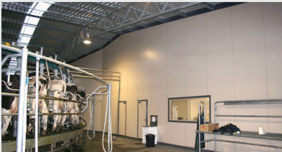
Internal walls seperating off milk vat room.
