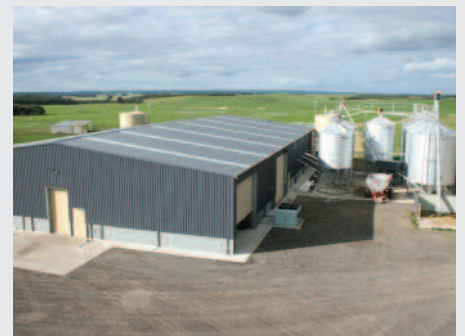
39m x 26m x 5m, with Ridgevent housing a 60 stand rotary.
